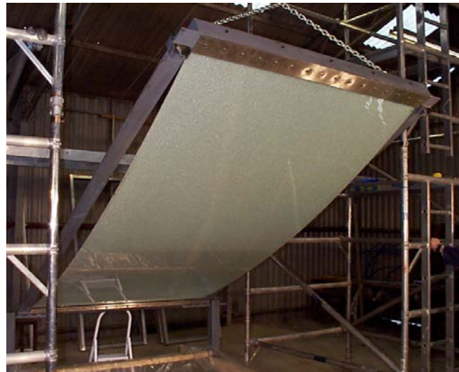
Overhead sloped glazing testing
